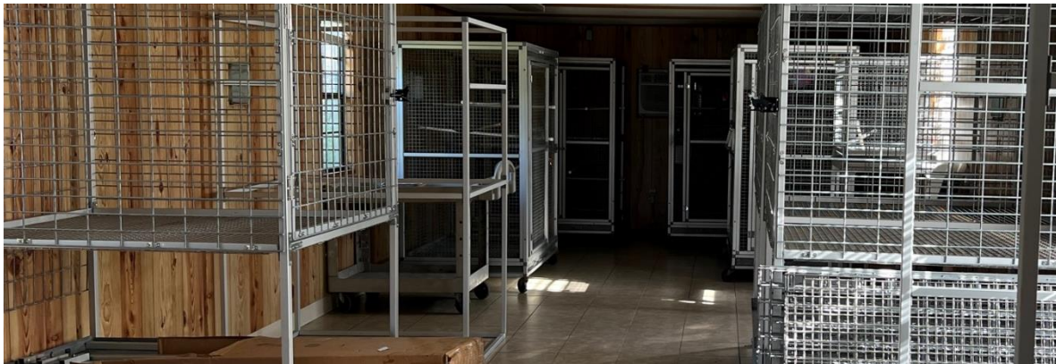
Constructing Capuchin Enclosures Inside Lollipop Guild
